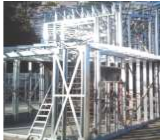
Cold-Formed Steel framing
